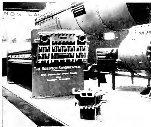
Fig. 2.—Showing Removable Front Cover.
